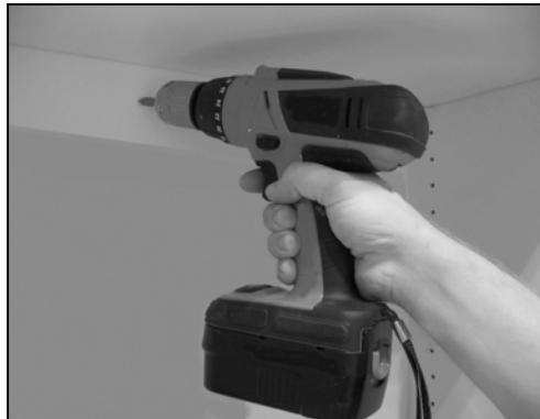
Secure plumb and level sections to wall.
